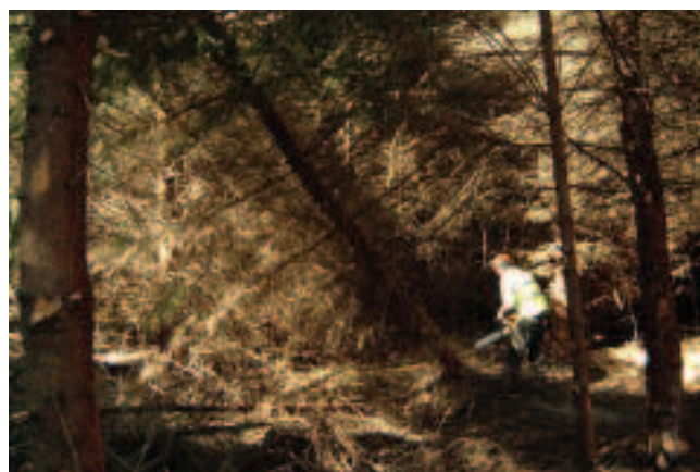
Felling trees in the line by chainsaw.
